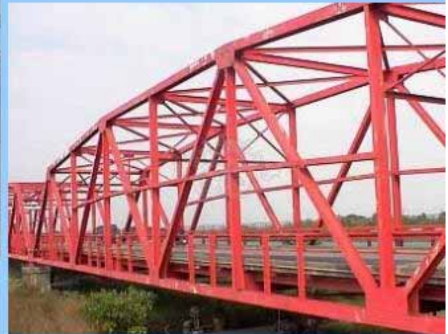
ShiLoh Steel Bridge since 1953
