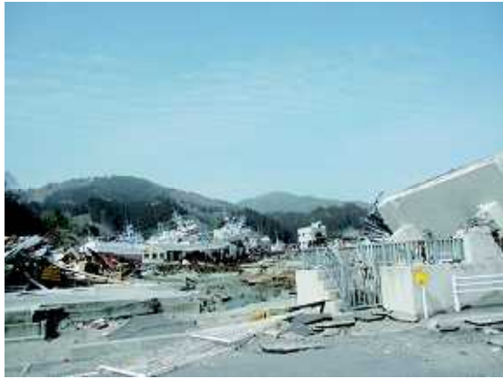
Photo 7 – The damage situation at the Shikaori District of Kesennuma City. Large fishing vessels and other things destroyed the protection line of the coastal levee, which is seen in the front of the photo, and were drifted deep onto the city area. In addition to the boats and ships, oil tanks, lumber, farming rafts, vehicles that were washed away by the tsunami are part of the factors that spread the devastating damage. (By Professor Fumihiko Imamura)
