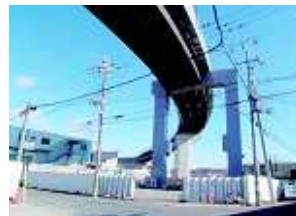
Photo 2: A steel fastening structure unifying the girder and the pier, and a narrow box girder was partially adopted.
