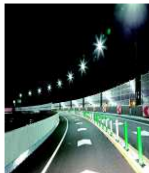
Photo 5: LED road lighting which was adopted for the arterial road of expressways for the first time in Japan.
