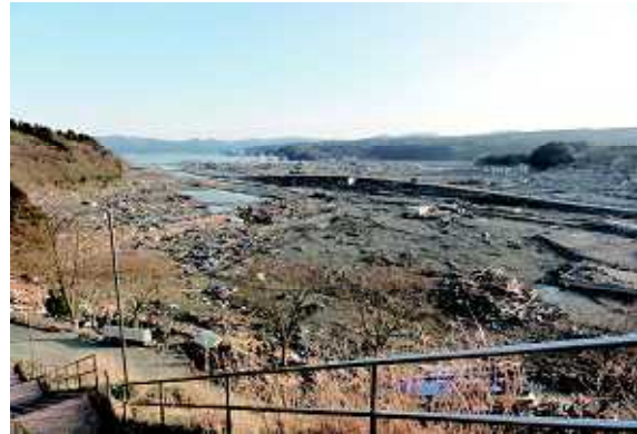
Photo 8 – Taken from the hilltop of Minami-sanriku-cho. Almost all the buildings were washed away except a number of reinforced concrete buildings on the beach. It was reported that the approximately 75cm-deep ground subsidence occurred in Minami-sariku-cho due to the earthquake. (By Shunichi Koshimura)
