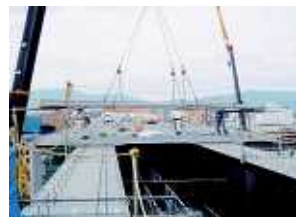
Photo 3: The erection of the bottom steel plates of the composite slab.
