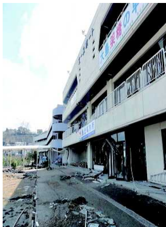
Photo 6 – A dock at the back of Kesennuma Bay (Minami-machi). The tsunami flooded up to the 2nd floor. It flooded up to the Kesennuma City Office. (By Shunichi Koshimura)
