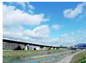
Photo 4: Unifying the girder height, considering the continuity since it passes along the Kamo-gawa River.
