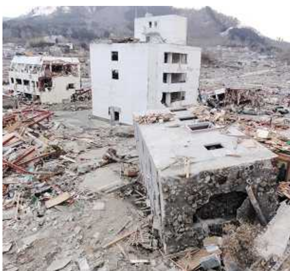
Photo 3 – A reinforced concrete building that fell down in Onagawa. It is considered that the bearing power of the piles was lost by the earthquake and it fell down by the tsunami which came subsequently. Until then concrete buildings had been believed to be able to withstand tsunamis. You can see an automobile which was drifted onto the roof of the building in the back. (Taken by Associate Prof. Shunichi Koshimura)
