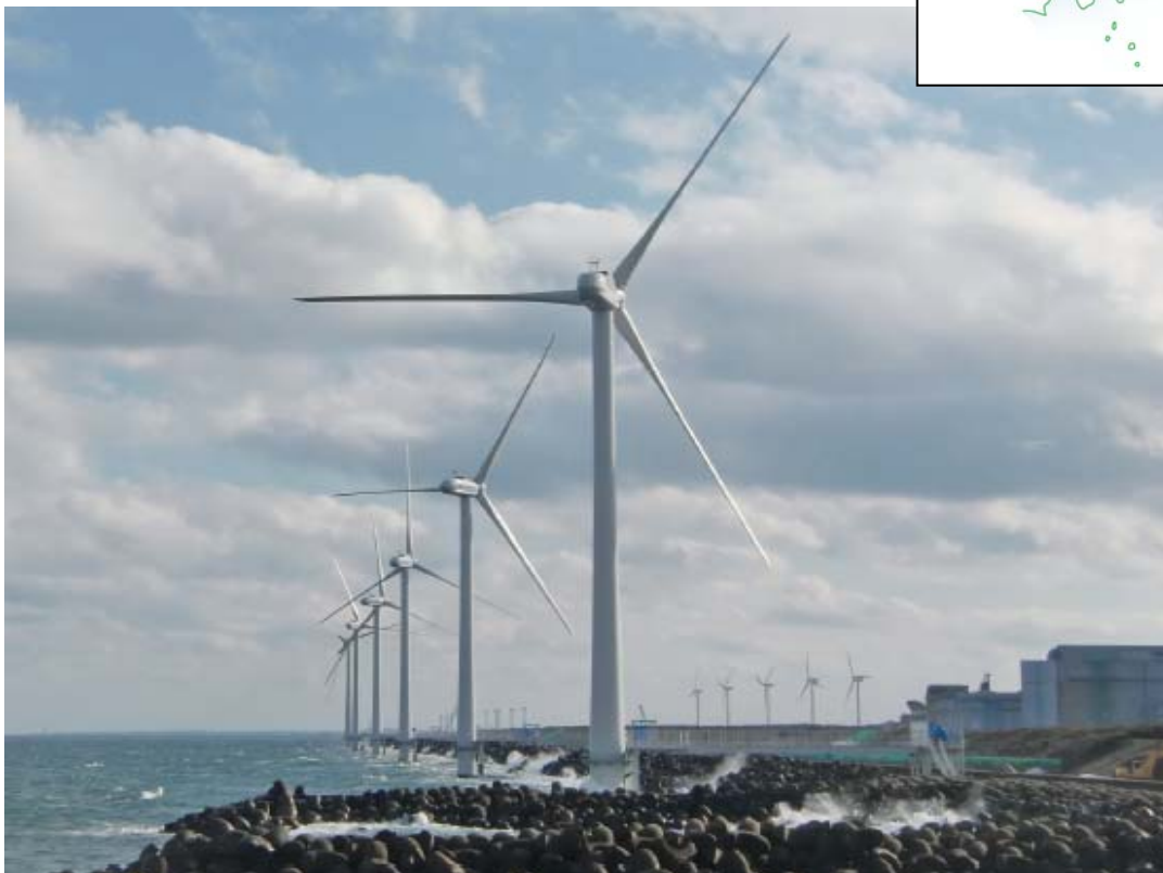
▲ Wind Power Kamisu (Photo taken from No. 1 wind turbine)
