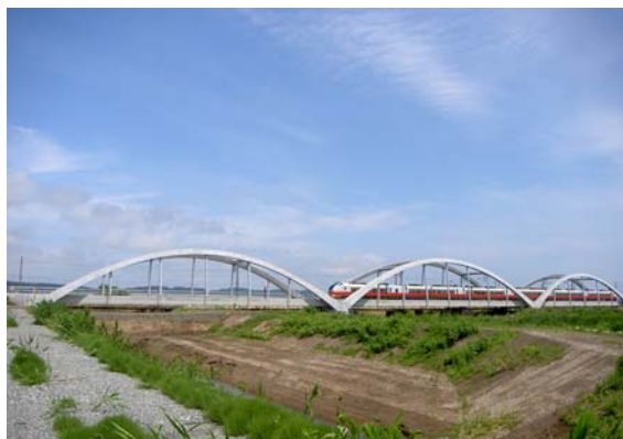
Tenmagawa Bridge (Aomori pref.)
