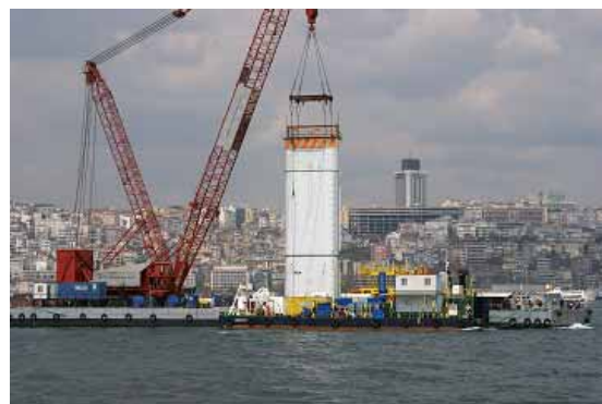
Photo.5 Temporary Access Shaft (Before Connection)
