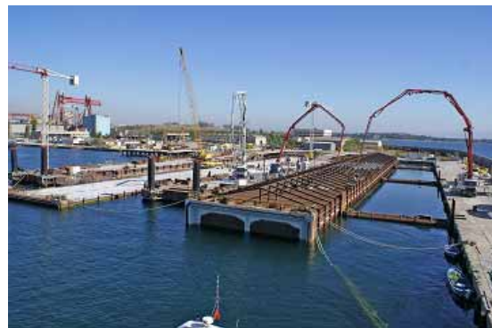
Photo.4 Element Construction on the sea (Floating Condition)
