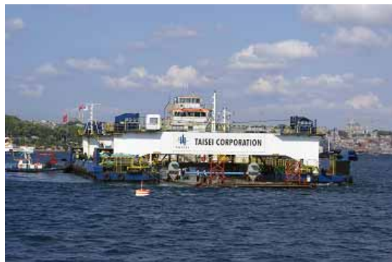
Photo.2 Placing Barge for Immersion
