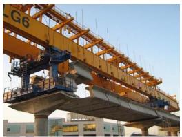
Viaduct Segments erected by a Launching Gantry
