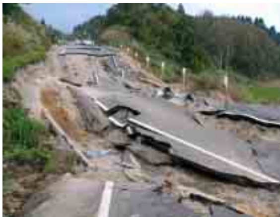
Photo 1- Collapsed National Road 117 in Ojiya City (by Dr. Kokushou)
