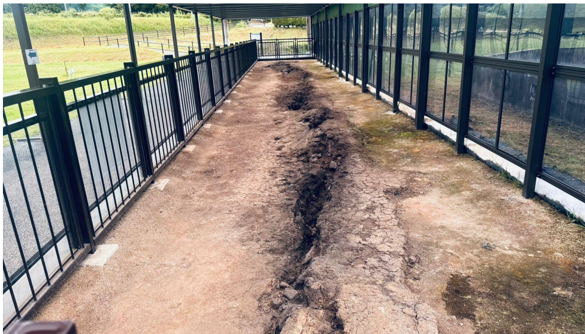
Photo 16: Visible fault line of the 2016 earthquakes
