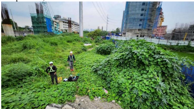
Figure 2.1.2.1 Estimated Pipeline alignment (center). Excavation site of affected property with water accumulation is visible on the right, and the Railway with transmission line on the left. Photo taken from the top of the backfill stockpile prior to removal.
