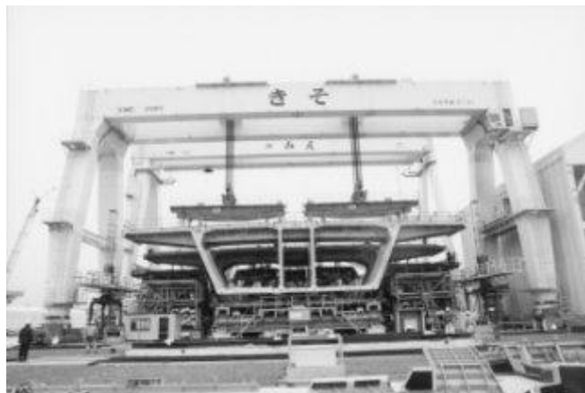
Precast Concrete Girder Segmen
