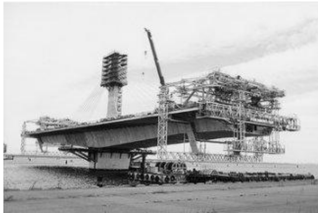
The Kiso River Bridge Under Construction
