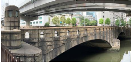
Tokiwa Bridge (Chuo-ku, Tokyo)
