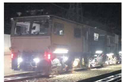
Fig. Track realignment using a multiple tie tamper
