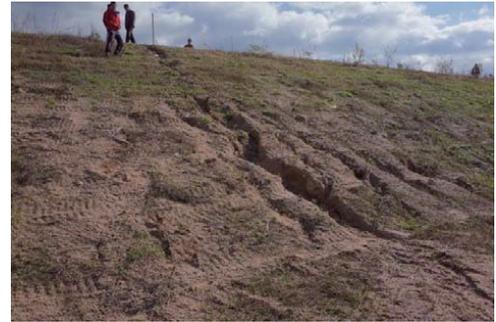
Fig. Erosion on the slope of a levee
