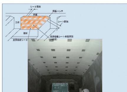
In the method of strengthening RC deck slabs using carbon fiber sheets, which are light and have excellent strength, during inspection of the deck slab, it is bonded in a lattice manner so that the underside of the deck slab can be seen
