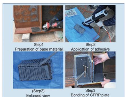
Method of strengthening corroded parts of steel members by bonding CFRP plate, which has superior constructability than strengthening using conventional steel plate backing plates
