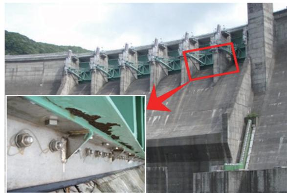
Fig. Corrosion in an emergency spillway (crest gate)
