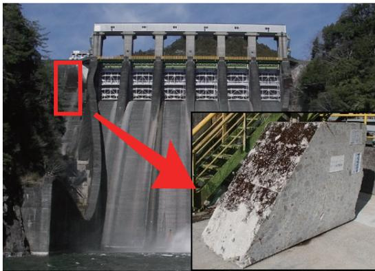
Fig. Concrete block from a dam excavated during dam re-development (sound even though more than 50 years had passed)
