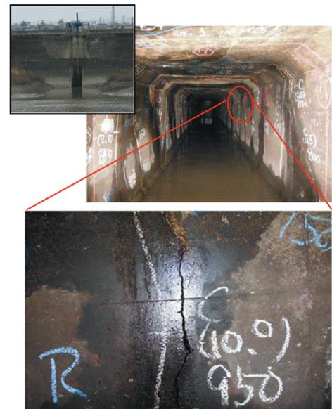
Fig. Crack in a sluice pipe
