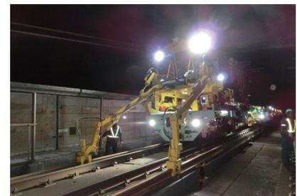
Mechanization of Shinkansen (continuous welded rail replacement)
