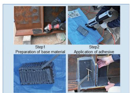
Method of strengthening corroded parts of steel members by bonding CFRP plate, which has superior constructability than strengthening using conventional steel plate backing plates
