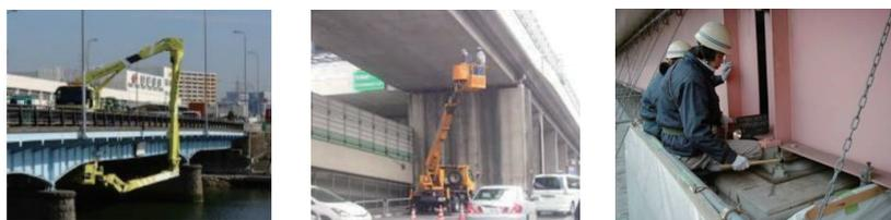
Fig. Close visual inspection of a bridge (bridge inspection vehicle, elevated working vehicle, construction scaffold)
