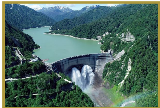
Civil Engineering Heritage: Kurobe Dam
