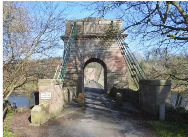
Masonry Tower and Anchorages on the Scotland Side of the Bridge
