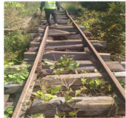
Photo 1 Seriously Damaged Track
