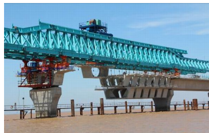
Photo 8 Segment hanging below the huge scale erection girder with hanging capacity of 1400t
