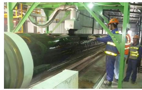
Photo 3 Coating SL compound in on-site fabrication facility to minimize the impact of weather and transportation
