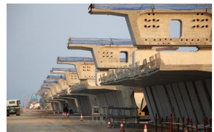
Photo 9 Precast pier head, preplaced segment waiting for erection girder
