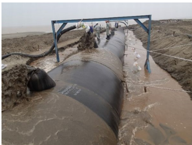
Photo 1 Slurry filling to Geotube (total length 24,000m)
