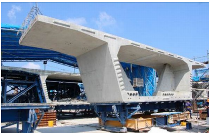
Photo 7 1405 nos of segment was fabricated by short line match cast method
