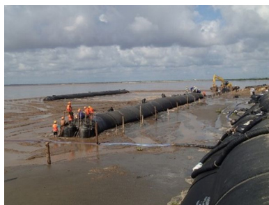
Photo 2 Laying lowest layer geotube during low tide
