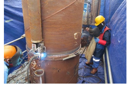
Photo 6 Executing site welding of upper and lower pile by 2 nos of automatic welding machine
