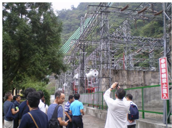
Takuan Hydroelectric Power Station at Sun Moon Lake, Central Taiwan, 748 m above sea level
