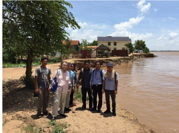
Slope Failure of Mekong Riverbank at Lerkdek District, Kandal Province, Cambodia (3 rd August 2017)
