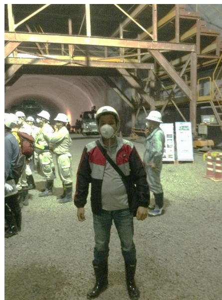
A Tunnel Construction Site in Hokkaido in 2014
