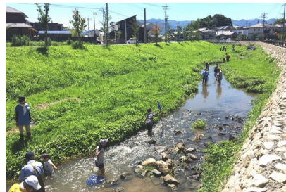
Stream restoration project in Kamisaigo River
