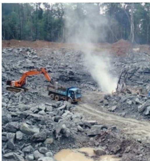
Collecting rough stones (stacking stones and drilling holes for blasting purposes)
