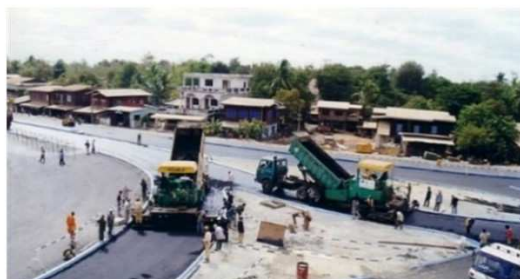
Paving of Seno Intersection
