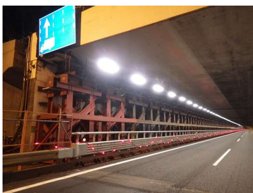
Photo 2 Installation of Temporary Supports
