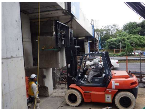
Photo 3 Transportation of Concrete Cut into Small Blocks
