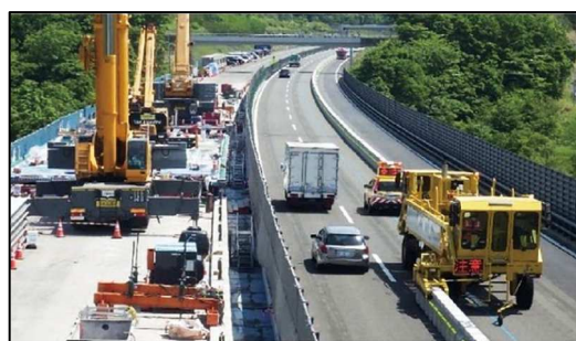
Photo 1 Changing Number of Traffic Lanes with Road Zipper System
