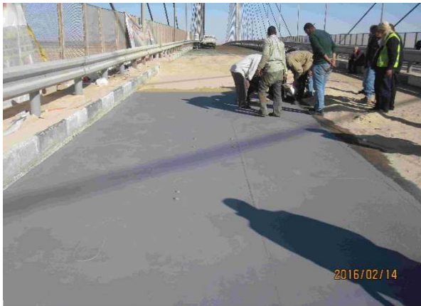
Sandblasting Treatment of Steel Deck Plate Surface
