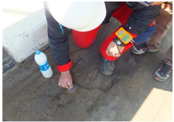
Measuring Reduction in Thickness of Steel Deck Plate
