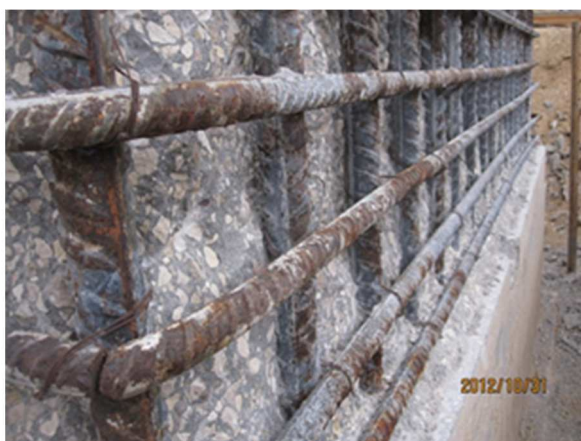
Rust on Piers
