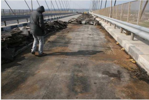
Rust on Surface of Steel Deck Plate (#2)
