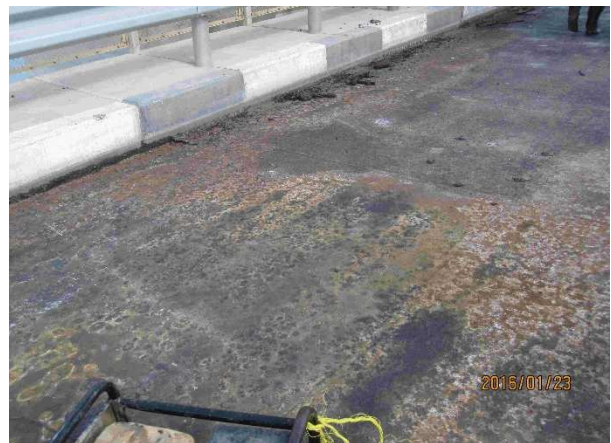
Rust on Surface of Steel Deck Plate (#1)
