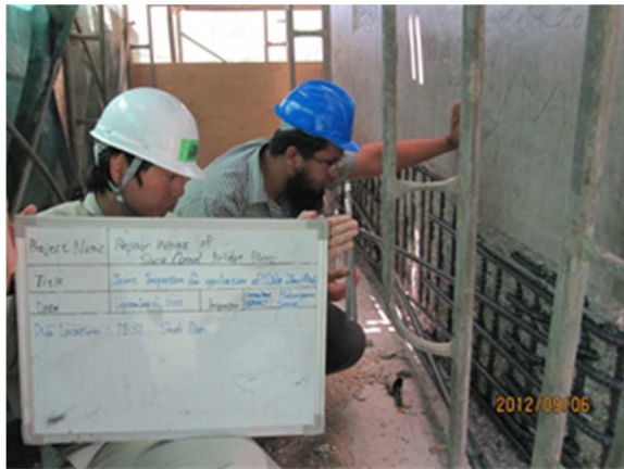
Egyptian Engineers Inspecting Japanese Company's Construction Work
