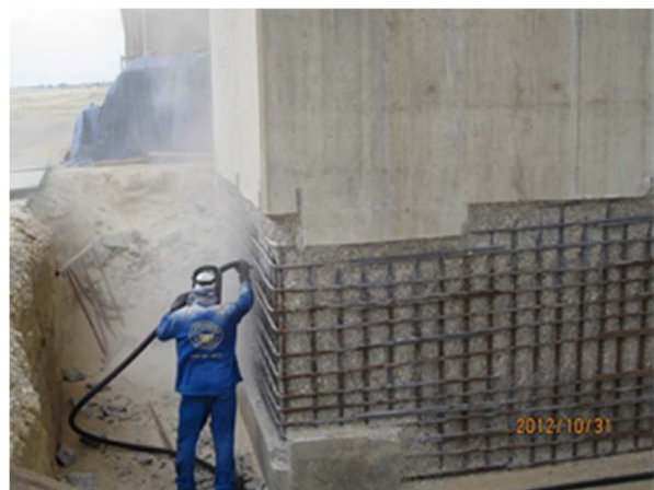
Removal of Rust on Reinforcing Steel Bars Rust on Piers
