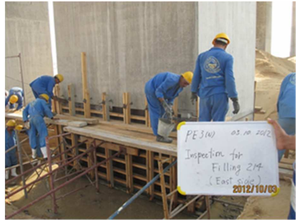
Filling of Repair Mortar
