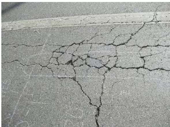
Cracks in Road Surface
