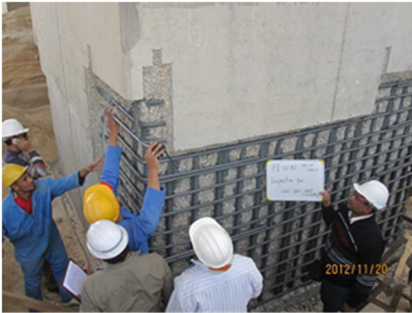
Egyptian Engineers Inspecting Rust Prevention Coating
