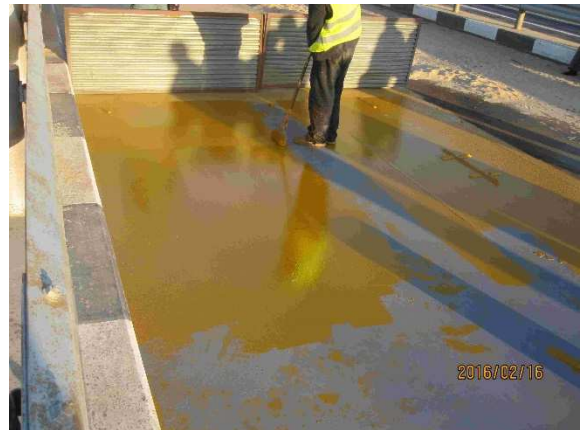
Applying Primer After Surface Treatment of Steel Deck Plate
