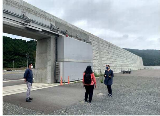
High Seawall as a Countermeasure to Protect the Surrounding Area, Built Along in Ogatsu Bay, Tohoku.
