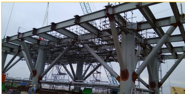
Fabrication of Superstructure of Jacket Type Jetty
