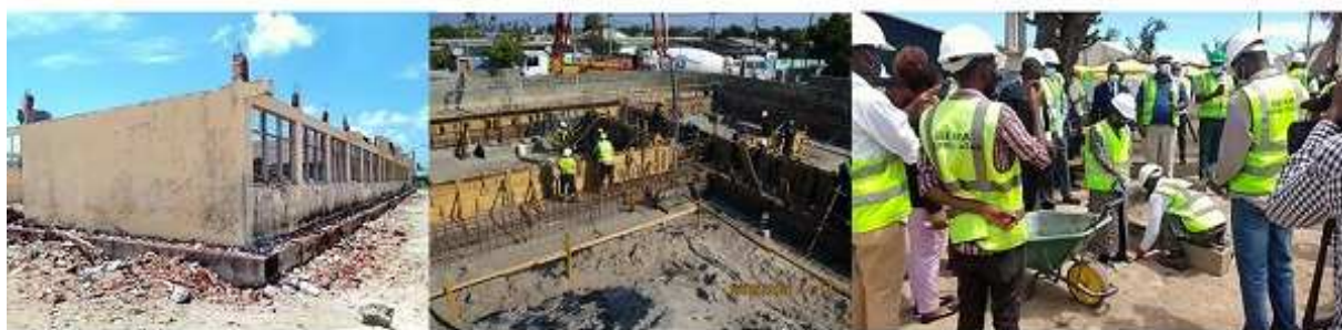
Recent Picture of Construction Work
