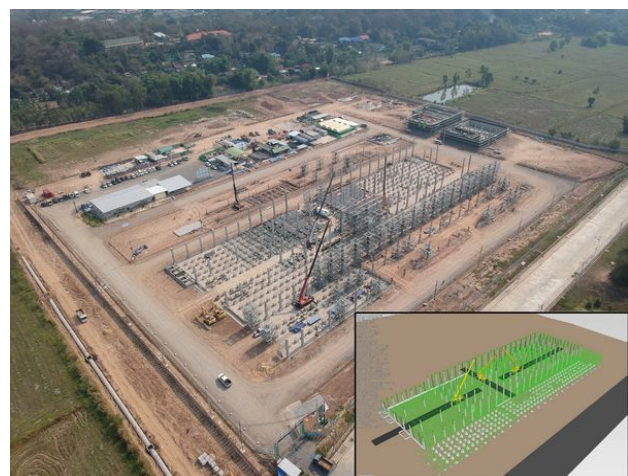
Photo 2: Working as a Project Director in Food and Cold Storage Factory Construction Project
