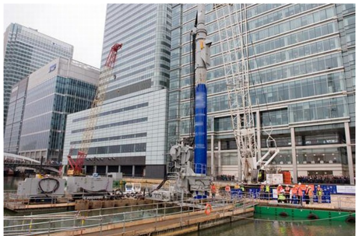
Photo 1: Tubular pile cofferdam was built to enable water retention at a depth of 10 meters.
