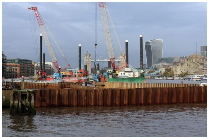
Photo 3: The twin Double Z sheet pile cofferdam project at the Thames
