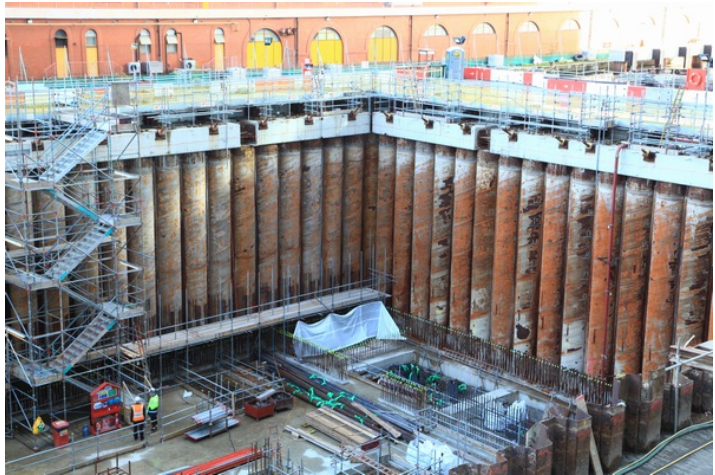
Photo 2: Inside of the cofferdam after discharging water
