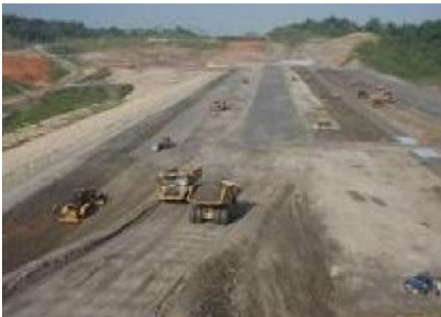
Overall view of building the embankment for Hushan Dam
