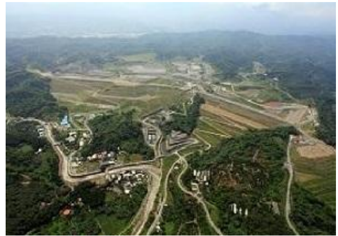
Aerial photograph after completion of Hushan Dam
