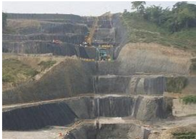
Construction of the continuous diaphragm wall on the left bank of a subsidiary dam
