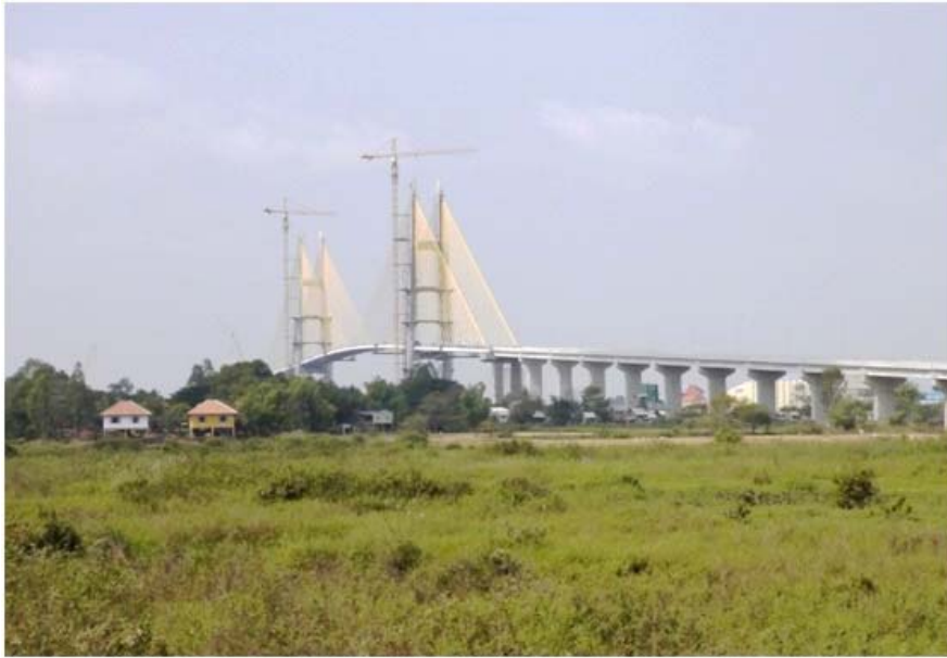
Photo 1. Neak Leoung Bridge in Cambodia under construction, which is implemented on an ODA grant-aid. The completion of the bridge will make significant contribution to the revitalization of economic activities in the area along the South Economic Corridor of the Greater MeKong Subregion.
