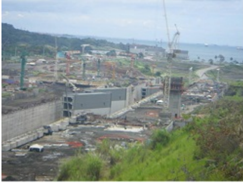
New Gatun Lock construction site on the Atlantic Ocean side
