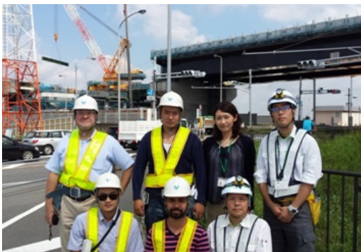
Observing construction work on the Shin-Katsushika Bridge of NEXCO East
