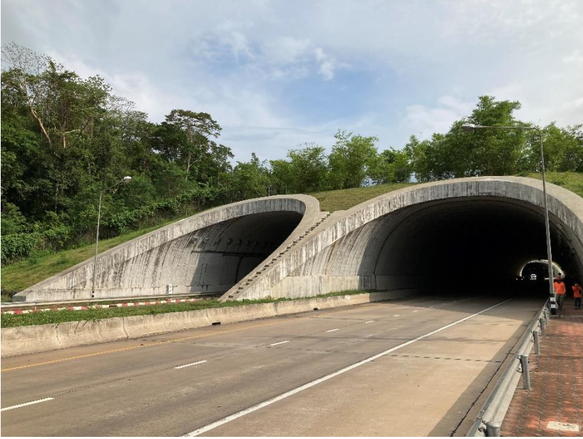
Road tunnel constructed on Highway 304 using cut-and-cover construction method
