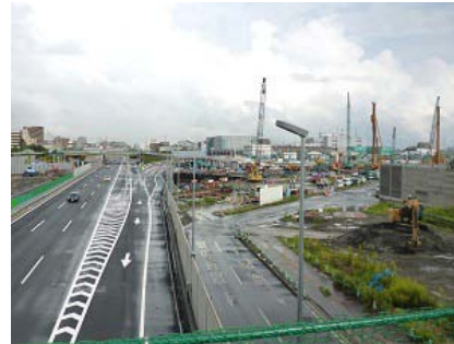
【Keiyo Junction】 A construction site in bird-view.
