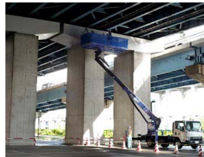
【Hamacho-minami Elevated Bridge】 Inspectors do inspection on the deck and piers on a lift
