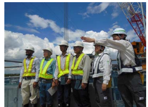
Shin-Katsushika Bridge by NEXCO EAST (Steel Superstructure Work)
