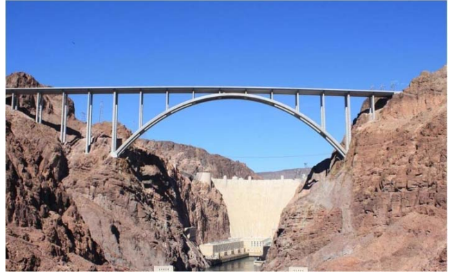
Fig.6 Colorado River Bridge
