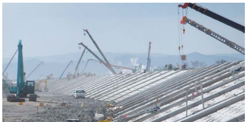
In a coastal area of southern Sendai, work is underway on the reconstruction of sea embankments. (Photo taken in March 2013; provided by the Kanto Regional Development Bureau.)
