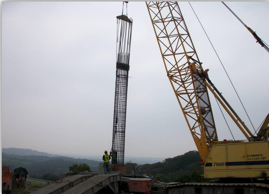
All casing concrete piles
