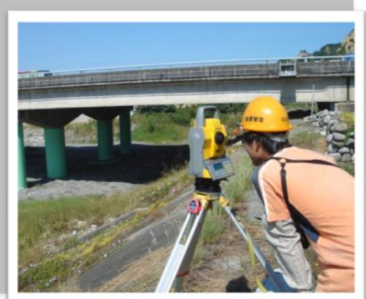
Riverbed cross-section measurements
