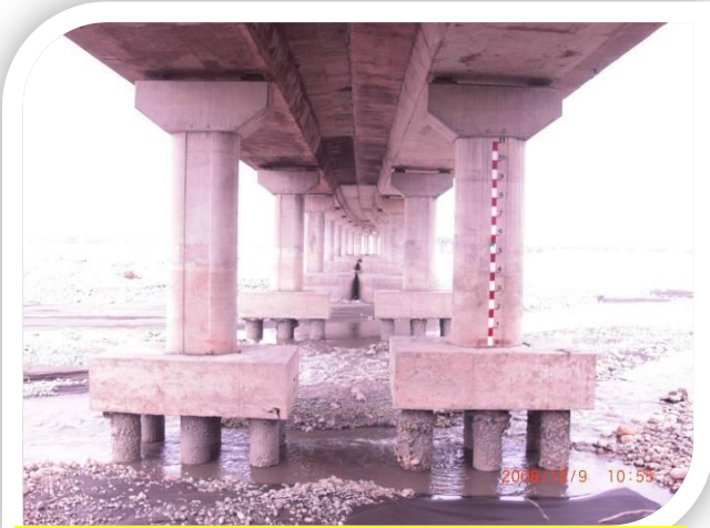
Pier base erosion
