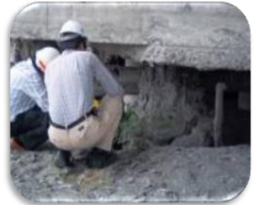
Pier base erosion
