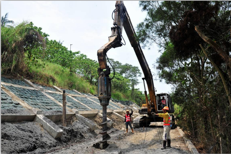
Retaining wall with piles
