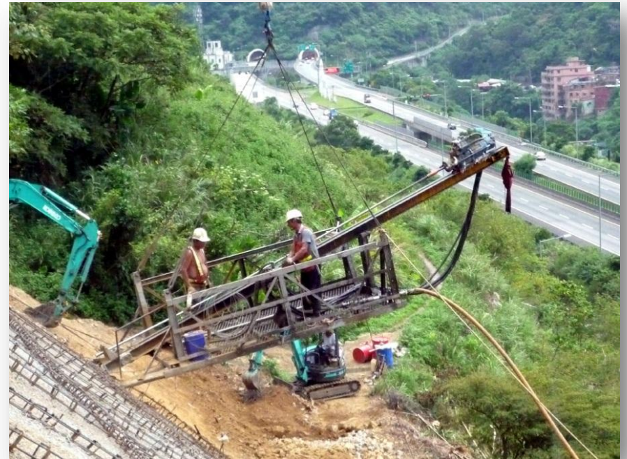
Rock anchors with shotcrete grids
