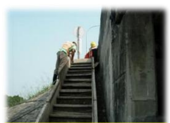
Additional maintenance ladder
