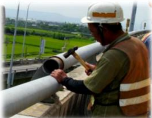
Bridge railing replacement
