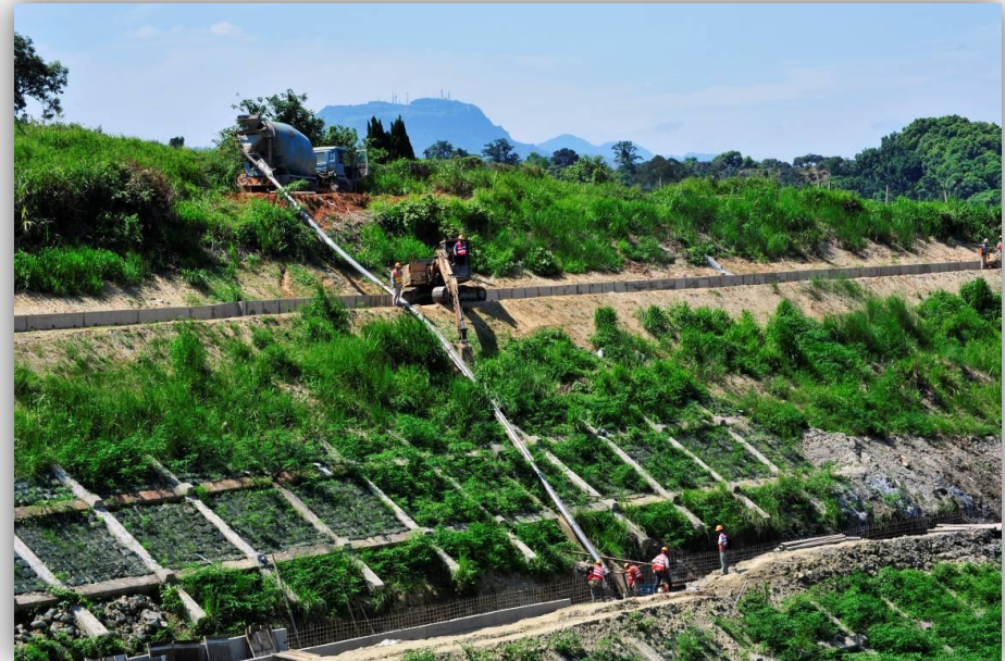
Berm ditch with mini-piles
