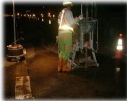
Grouting in bridge concrete slab
