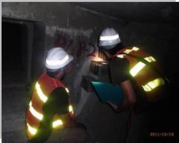
Box girder internal
