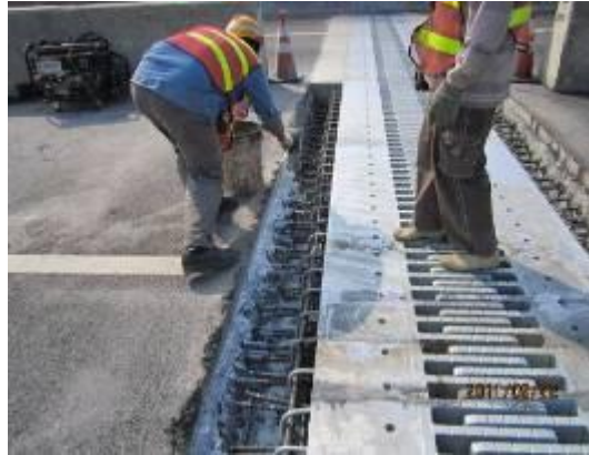
Expansion joint replacement
