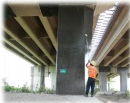
Pier steel plate paint
