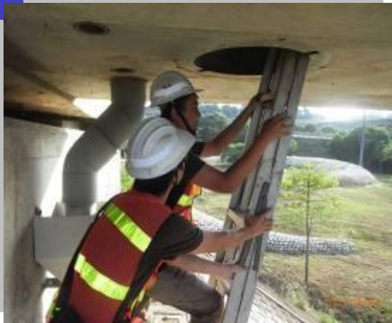
Box girder internal
