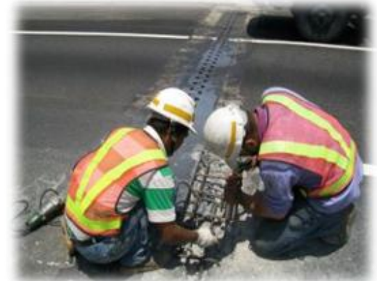
Repair expansion joint
