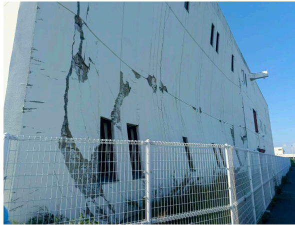
Structurally damaged wall of old warehouse building of Minami-Gamo Wastewater Treatment Plant.
