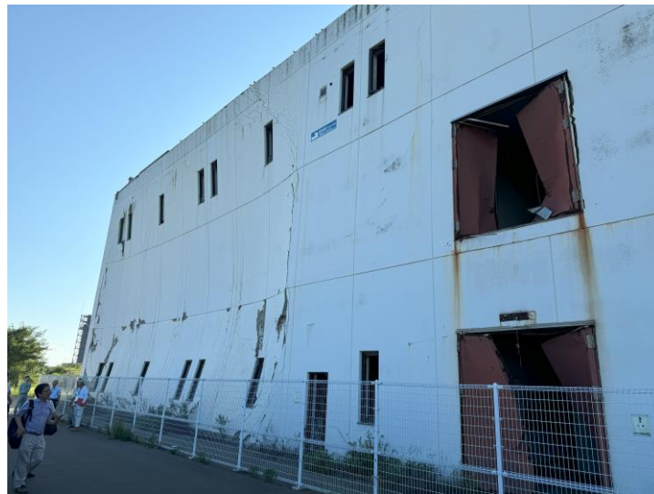
Figure 16. Damage hit by 10.4m height Tsunami wave at Minami Gamo Wastewater Treatment Plant
