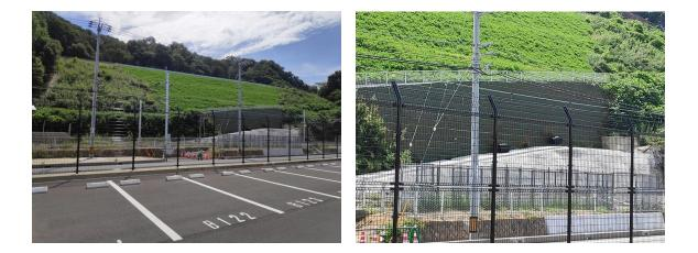
restoration, the slope was stabilized by slope cutting and compaction. Land of highway 31 provided as working place and temporary sediment storage during the sediment removal process and detour road was used as approach road. Road construction was finished in 2 months ahead of schedule and JR Kure line resumed operation on September 2019.
