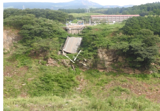
Figure 22, 23 The collapse of Aso Bridge
