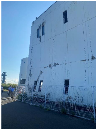
Fig.7. The 3rd pumping building with the wall curved by the tsunami
