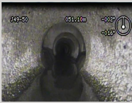
Concrete Corrosion/Aggregate Exposure
