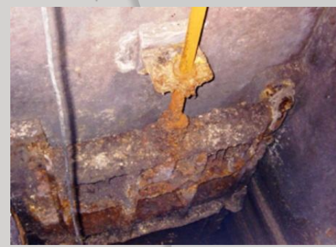
Ingress Gate difficult to open/close
