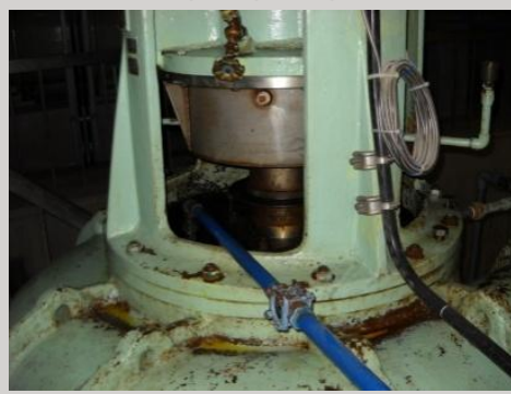
Damaged Bearings at Heavy-duty Pump
