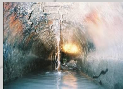
Underground Water Leak-in
