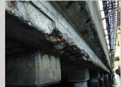
Flaking Caused by Rebar Corrosion
