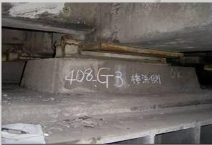
Corroded Bearing
