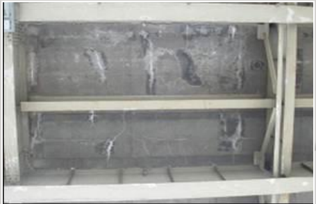
Cracks on Slab
