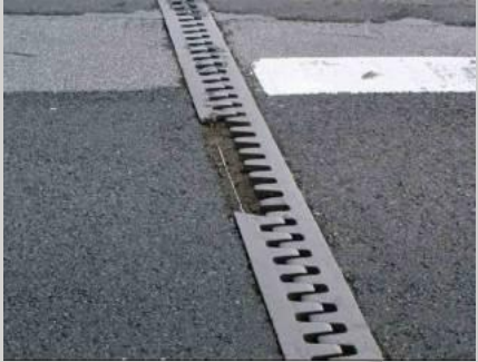
Broken Joint
