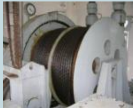
Gate wire rope
