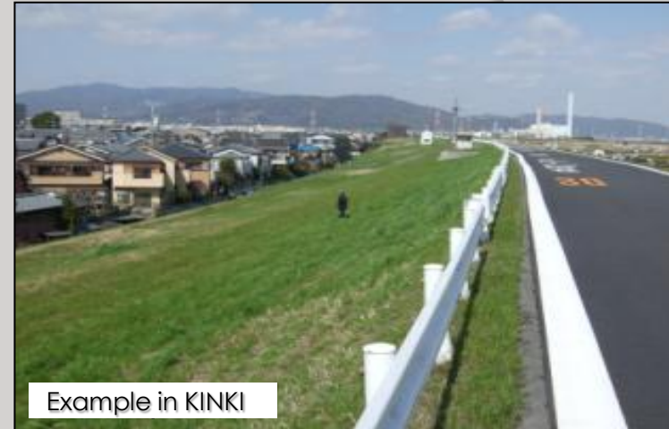
Bank Top higher than Houses
