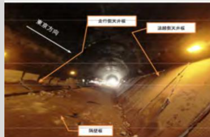
Fall of Ceiling/Bulkhead Boards at Sasago Tunnel, Japan
