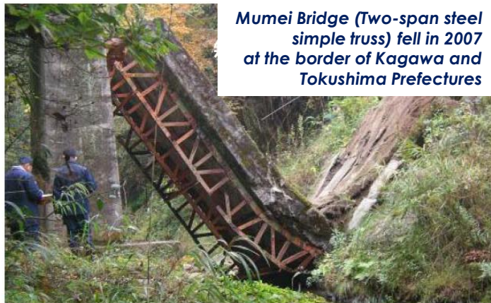
Damage examples from infrastructure aging
