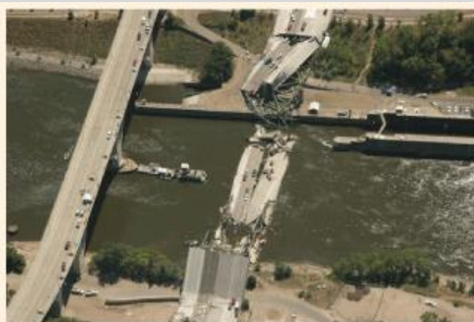
Collapse of Bridge in Minnesota
