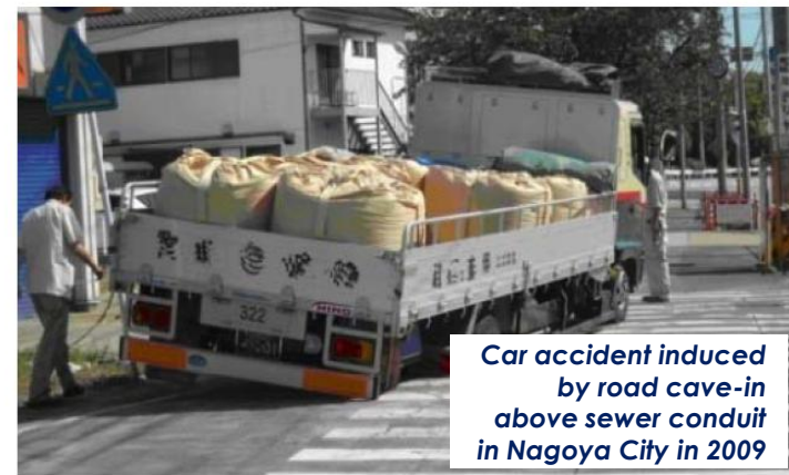
Damage examples from infrastructure aging
