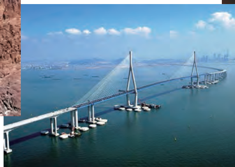
Incheon Bridge, Korea
