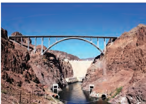
Colorado River Bridge, USA
