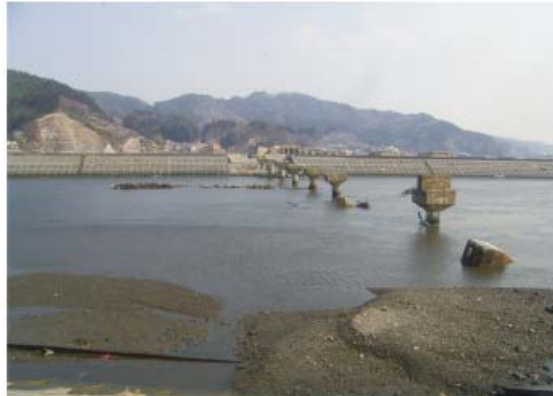
Photo 9: A bridge girder washout by the tsunami (Yamada Line, Kirikiri – Otsuchi)
