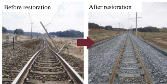
Photo 8: Failure of an embankment slope (Tohoku Main Line, Umegasawa – Nitta)
