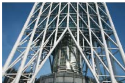
Photo 2: Inside of the central pillar under construction
