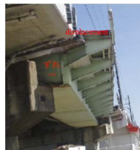
Photo 6: Bridge girder displacement (Kashima-Jingu Station, Kashima Line)
