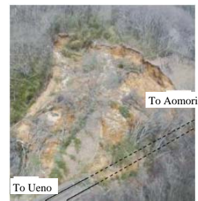
Photo 7: Collapse of an excavated slope (Tohoku Main Line, Toyohara – Shirasaka)
