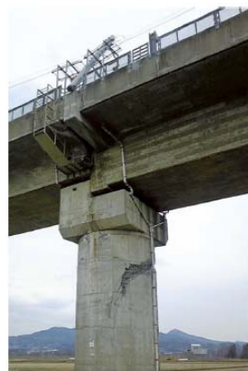
Photo 2: Damage on a bridge pier (Ichinoseki – Mizusawa-esashi)
