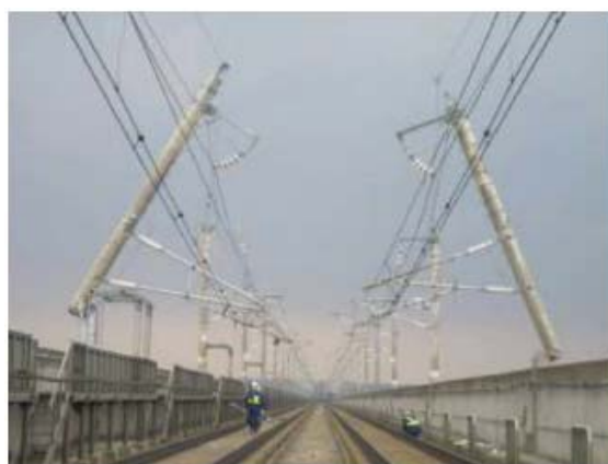
Photo 5: Damages on the power poles (Mizusawa-esashi – Kitagami)
