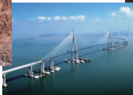
Incheon Bridge, Korea
