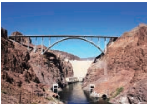
Colorado River Bridge, USA
